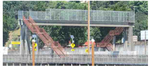
Existing Pedestrian Bridge over BNSF lines at Kalama
