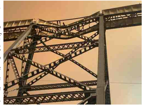
Photos of fire damaged Dry Canyon Bridge Viaduct. Photos courtesy of Union Pacific Railroad.
