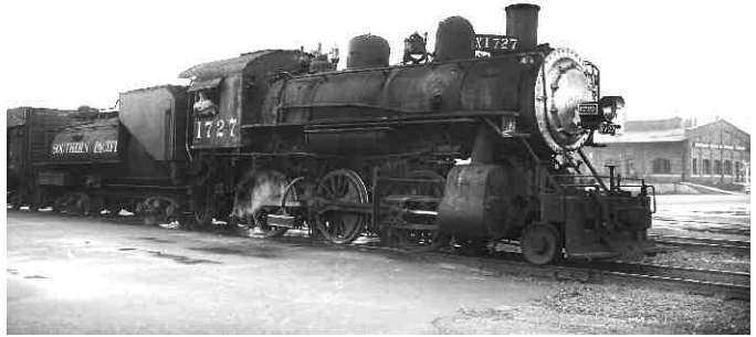
Dunsmuir's future Fresno Mallet #1727 is seen in service at Fresno, California on December 7, 1955. The doughty 2-6-0 has already given its owner 54 years of service at the time of this photo, and is still going strong. Photo from the collection of Kenneth G. Johnsen.
