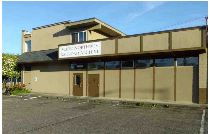
A new photo of the northside of the Archive showing the new awning to the left of the front doors. The awning was added to route rain water away from the building and increase the protection of our collections. The front of the Archive is only lite by the sun for this photo in mid-June of each year.
