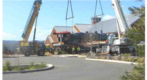
Boiler being placed on frame with "pusher in place"
