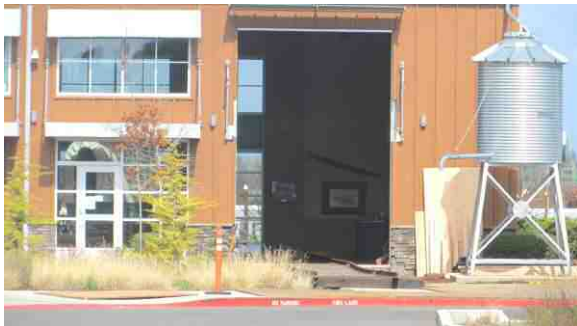
Port of Kalama office building with rails in place
