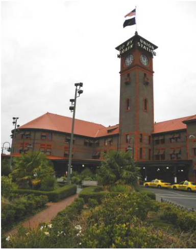
View of Area in Front of Station
