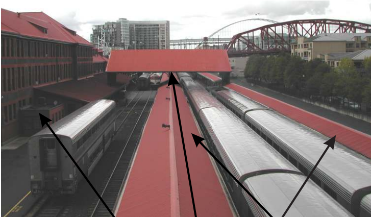
View of the Nursery (far left), High Shed and Platform Canopies
