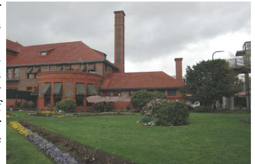
View of Area in Front Right of Station
