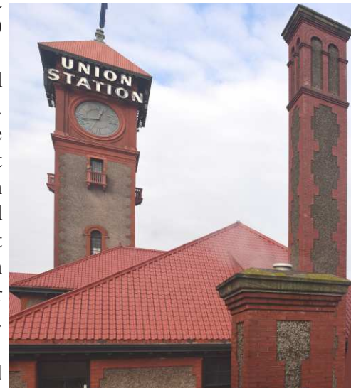
Detail of Roof, Brickwork and Stucco on Portland Union Station
