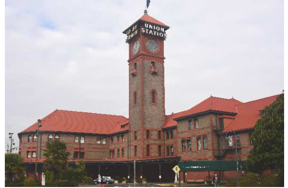
Front Entry to Portland Union Station
