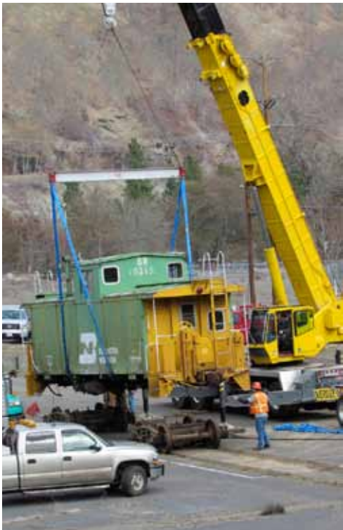
Above: The caboose arrives in Klickitat on a lowboy supplied by Redmond Heavy Hauling. Left: The caboose was carefully lifted from the lowboy and placed on its trucks. Accurately dropping a railcar on its centerpins is no easy task. (Photos by Allie Spino)
