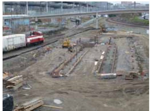
Right: At this point, the piling was in and the forms were being set for the floor under the tracks. (February 24 photo by Arlen Sheldrake)
