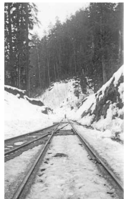
This view of the vacant trackage at Wedeburg shows that the Tillamook line received its share of snow in the winter. The high elevation of the railroad over the hills to the coast resulted in much inclement weather. Photo, PNWC collection
