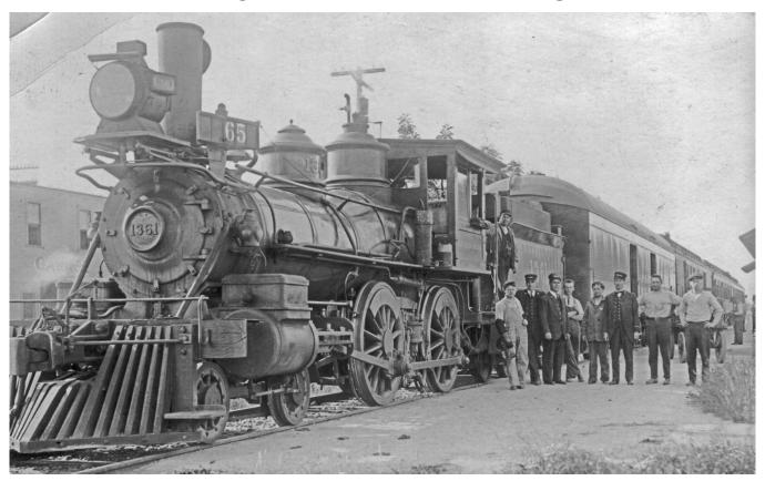
Above: Espee's #1361 was a 4-4-0 outshopped by Baldwin in 1883. She originally carried #28 on the Oregon and California. From 1909 to 1911, the locomotive was leased to the Astoria and Columbia River. After its return, the Southern Pacific ran the engine until its retirement in 1917. #1361 was scrapped at Brooklyn in 1920.
