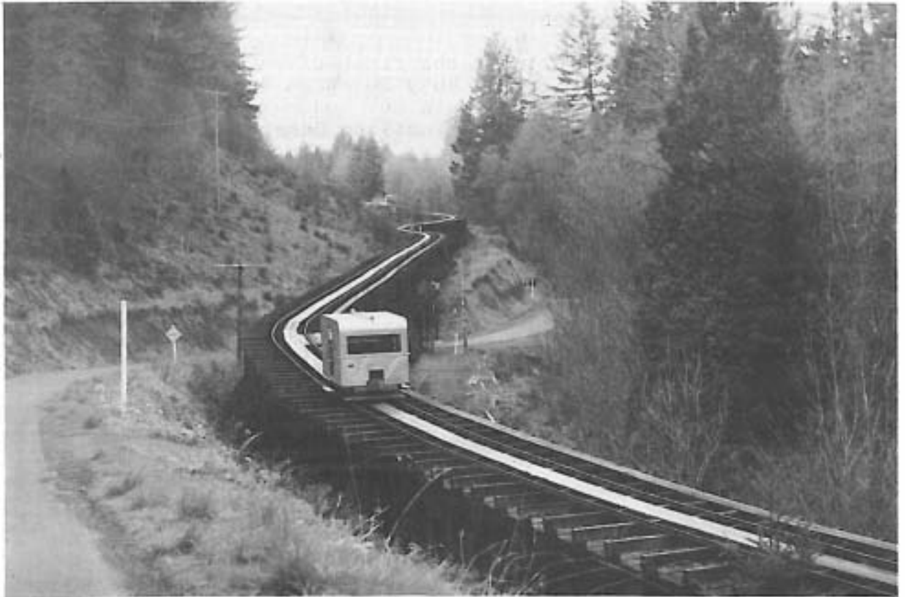
Motor car on Portland General Electric Company flume railroad near Roslyn Lake. Terminal of railroad is in center background. Photo by Chas W Storz, jr - 28 MAR 70.
