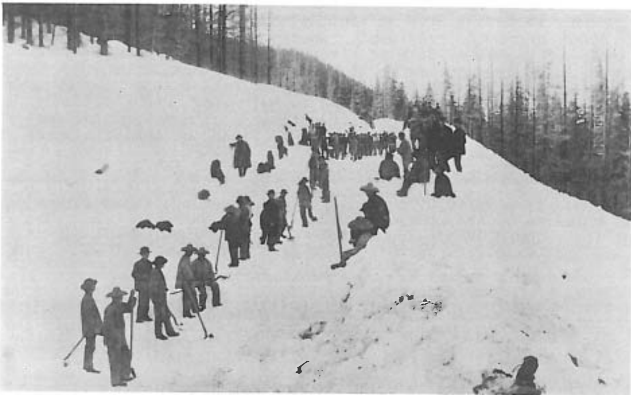
Chinese laborers shoveling snow for Northern Pacific track-laying crews near the summit of the Cascade Range in 1886. NP trains crossed this barrier by means of switchbacks prior to completion of the "Stampede Tunnel".
